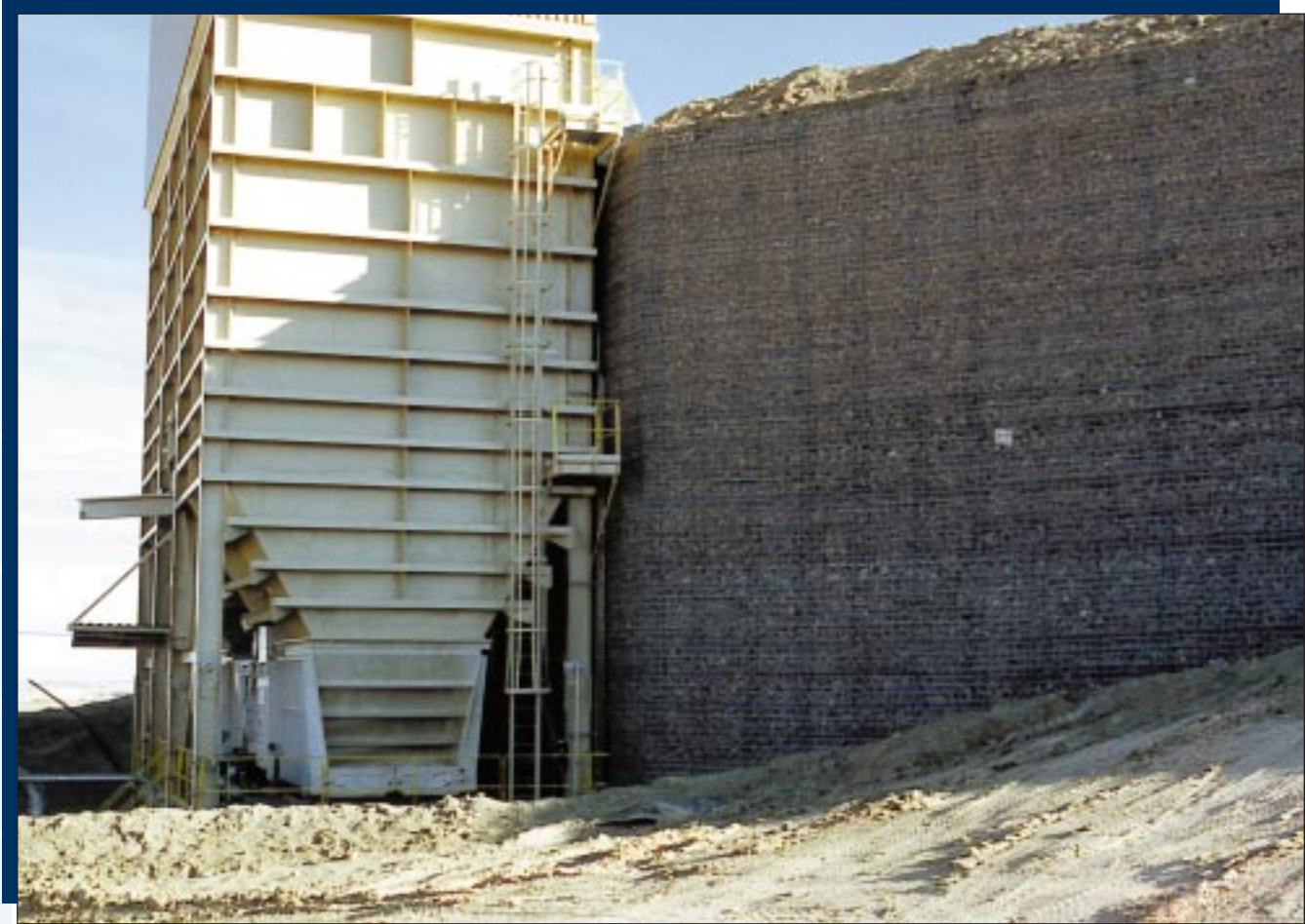
Permanent 18m tall Terratrel wire-faced head walls
