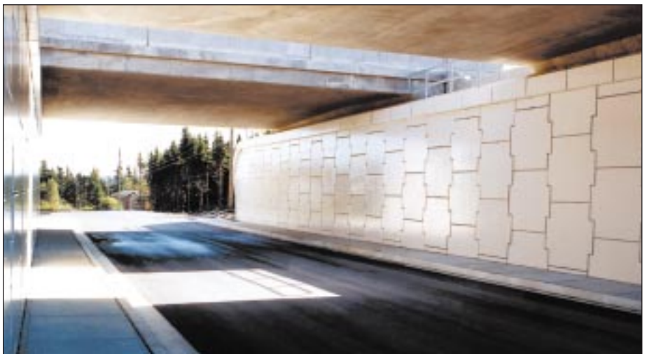
With the application of an anti-graffiti finish the Reinforced Earth Abutment wall for the Groves Road Overpass exhibits a brilliant and uniform finish.
