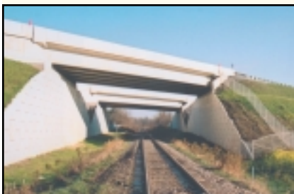
True Abutment wall for 407 ETR over CPR Havelock rail line.
