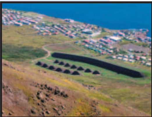
View from mountain slope to Neskaupstaður harbour, showing face of main dam with splitter walls in the foreground.
