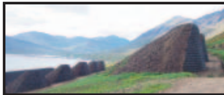
Completed TerraTrel splitter walls.
