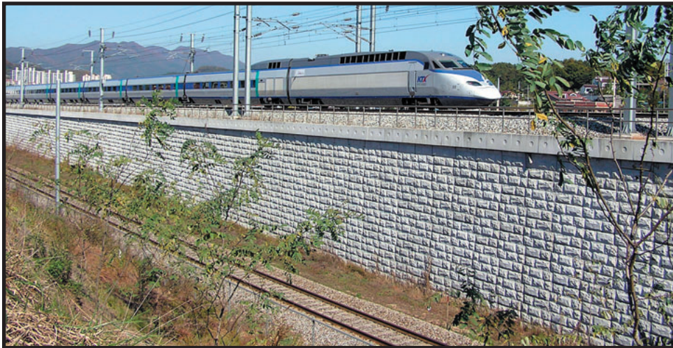
TerraClass panels with Ashlar Stone finish: 5,600m 2 (60,278 ft 2 ) x 10.5m (34.5ft) maximum height walls.
